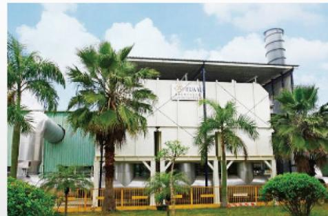
Regenerative Thermal Oxidation Production Line (RTO) is a common technology used for air pollution control in various industrial processes. RTO is used to treat volatile organic compounds (VOCs) and hazardous air pollutants (HAPs) emitted from industrial processes.
